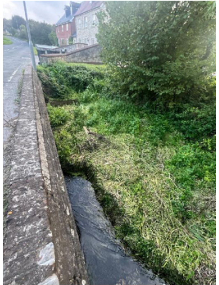
Photos to show the amount of weed still blocking Bridge 1 on The Moor, hindering fluvial flow
