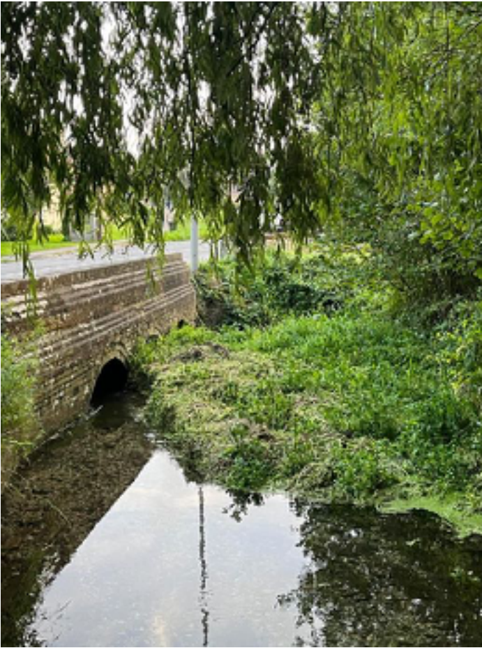
Photos to show the amount of weed still blocking Bridge 1 on The Moor, hindering fluvial flow
